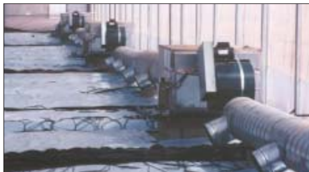
Multi-Duct System being installed for a vegetable production greenhouse in Mexico.
